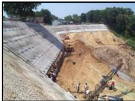
Fig-14 Soil Nailing
